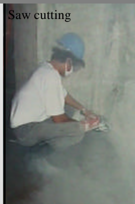
Saw cut repairs
