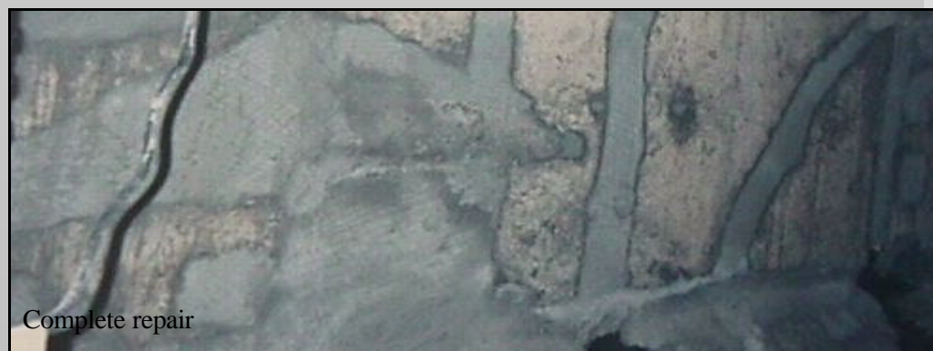
Base / waterproof repair complete
