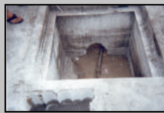
Pilot Bore Arrival Pit
