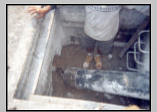
Back Reaming and Pull Back
