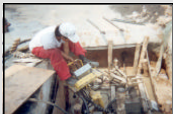
Drilling of Pilot Bore from Launch Pit
